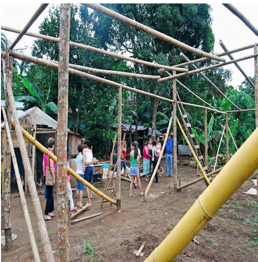
Construction of community greenhouse
