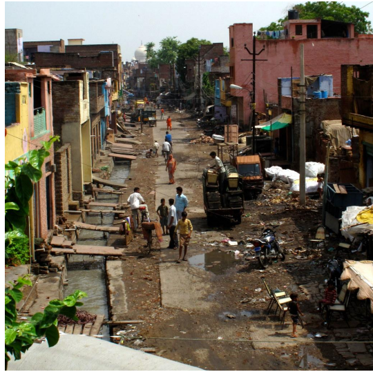
In Agra, open sewage ditches line the streets, threatening local water systems.
