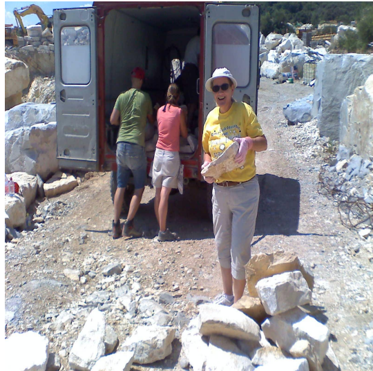
Gathering stones from the quarry to be used on the wall repair.
