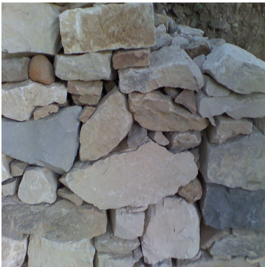
A section of the wall in progress: Look - no mortar!
