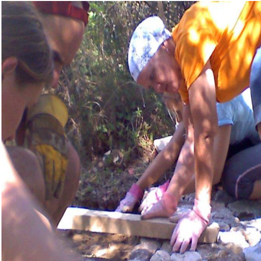
Repairing and re-paving a section of a thousand-year-old path.
