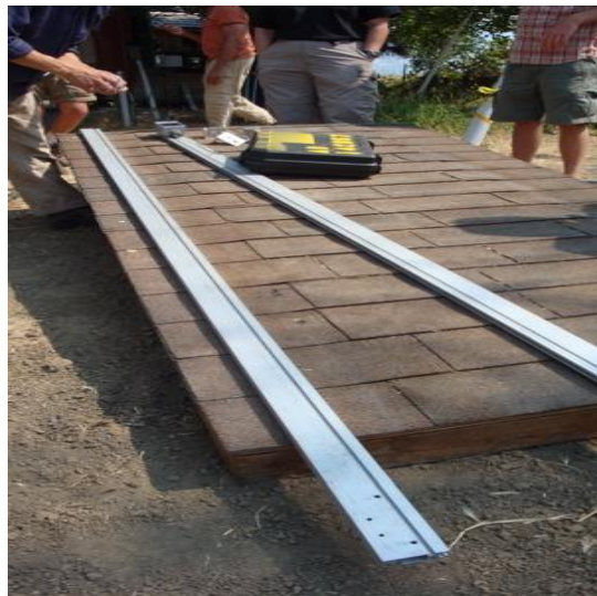
Simulated roof top and hardware to affix solar panels
